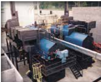
TWIN 600 BHP Hardwood veneer plant, Steam vats and coil dryer heat application.
