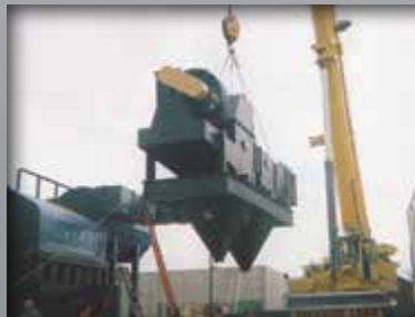
TWIN ASH COLLECTORS Primary and Secondary Modular Units being lifted into place.
