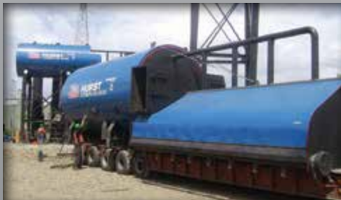
TWIN 1200 BHP “Super Heated” 450 psi Erected in Dominican Republic.
