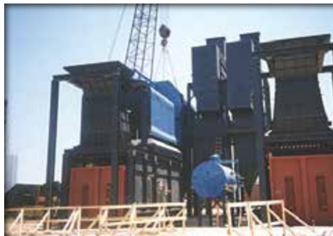
TWIN 1200 BHP 450 PSI Super Heated
