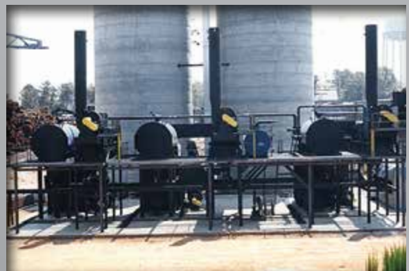
Triple 600 BHP w/ Silo Fuel Storage
