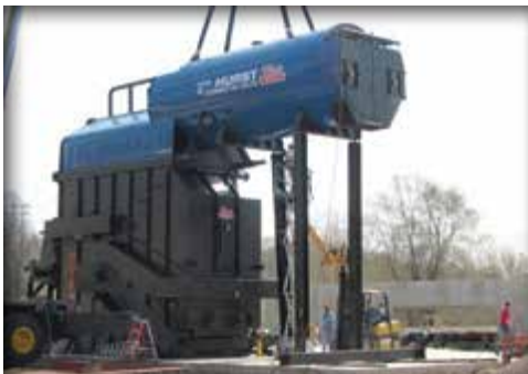
1500 BHP 1500 BHP, 250 PSI design being erected in Wisconsin. This assembly is shipped in 3 large modular pieces for a cost saving installation.
