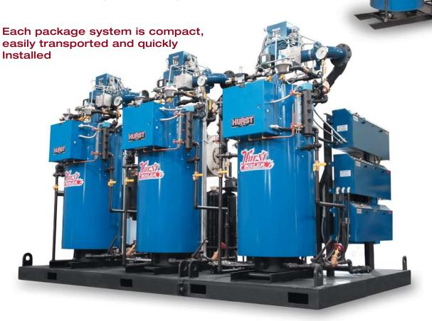
Hurst Boiler offers premium customized boiler skid packages for all types of steam and hot water boiler applications
