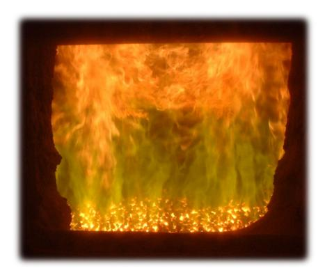
This is another great photograph of the inside of a furnace. As the volatiles are released from the fuel, they meet streams of high pressurized air from the over-fire jets. This turbulent mixing of air and volatile gasses completes the combustion process, releasing heat to be transferred within the boiler.
