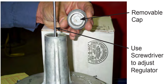
Figure E – 9 Main Gas Pressure Regulator Adjustment
