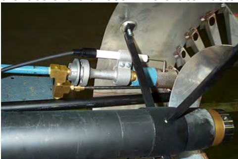
Figure B-11 Pilot and Scanner Sight Tube
