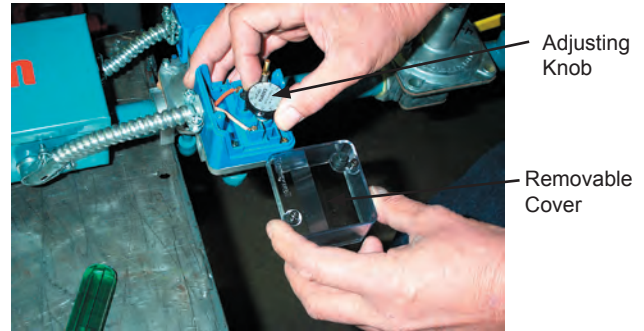
Figure E – 10 Gas Pressure Switch Adjustment
