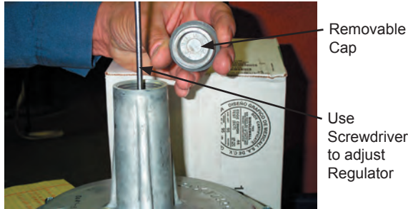
Figure E – 9 Main Gas Pressure Regulator Adjustment
